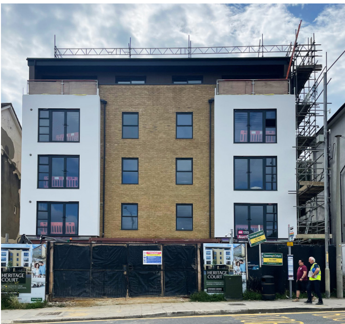
18. Watertight Construction Site, June 2023
