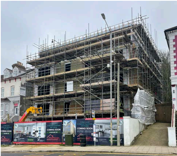
17. Construction Site, August 2022
