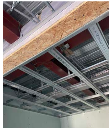
21. Ceiling installation, September 2023
